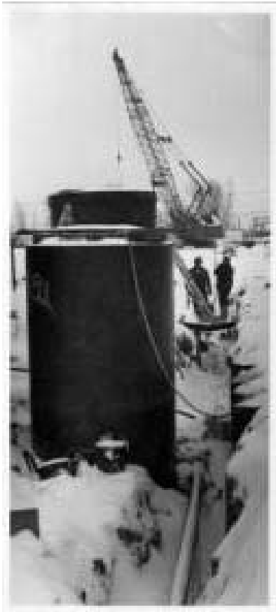
Remediation work at Love Canal showing large containment tanks and crane
